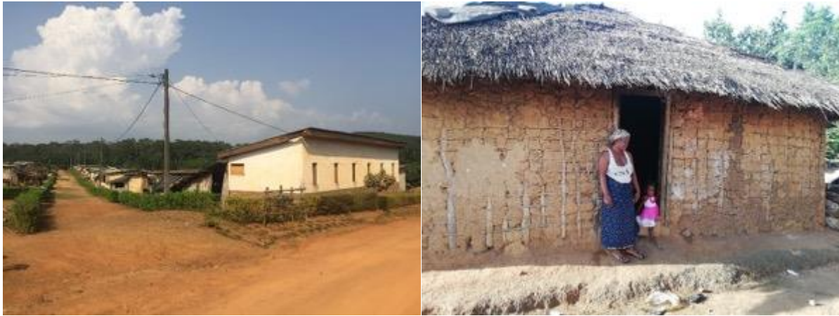
Figure 7–10: Brick structures at Kako (left) and typical mud, wood and raffia houses from a neighbouring village (right)
